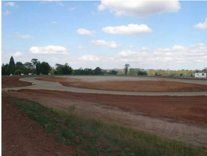
Forest Rd Site preparation Dec 2007
