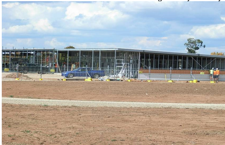
Framing Stage April 2008
