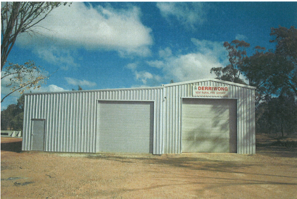
Completed extensions at Derriwong
