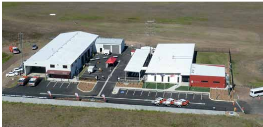
The new Northern Rivers Fire Control Centre Complex seen from the air. Photo by Steve Nixon
