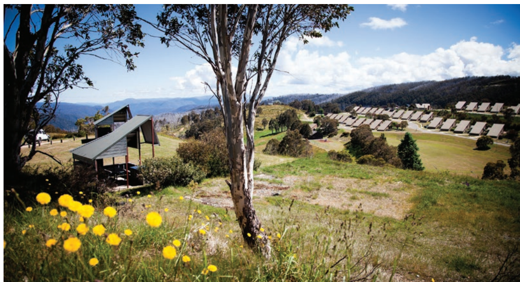
LEFT: A basic architectural design of all the buildings in the town to cater for effects from the winter snow added several benefits to managing property hazards for bush fire protection. For example buildings do not have guttering, the angle of roof pitch is very steep and resists embers and ash settling on roofs, and the roofing iron is continuous from top to bottom with no gaps. The landscaped area around the houses complex is minimal and consists mainly of well maintained lawns, paths and featured rock walls.
