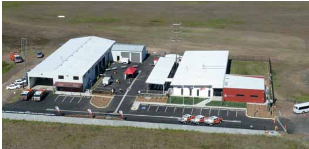
The new Northern Rivers Fire Control Centre Complex seen from the air. Photo by Steve Nixon
