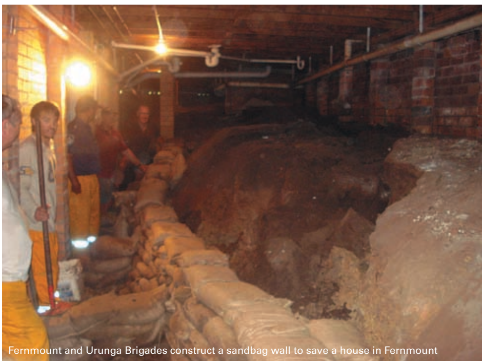
After their station was badly damaged in the floods, the Urunga NSW Fire Brigades move into Urunga RFS station
