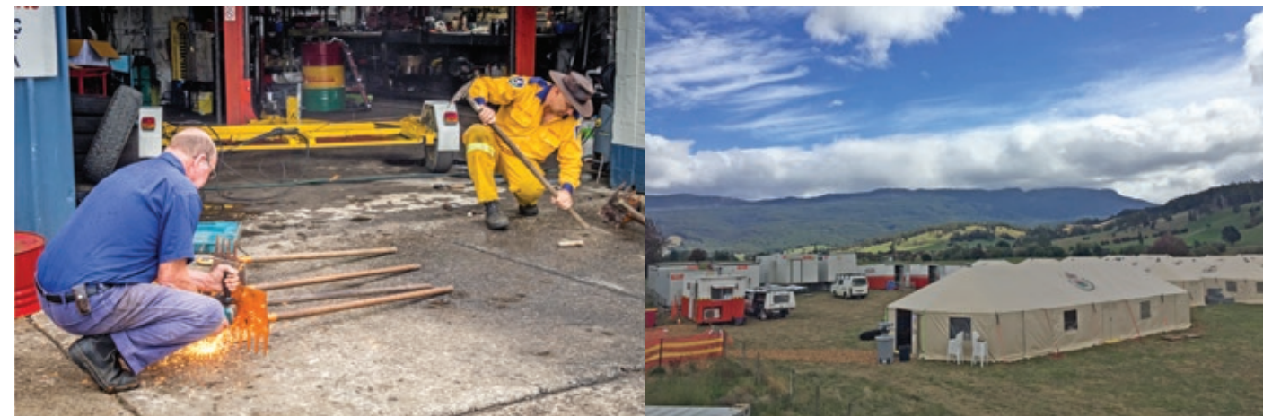
ABOVE LEFT: Bruce Coomer, Blue Mountains RAFT, and the owner of the service station at Mole Creek R&D Motors, modifying the rake hoes. Nicole Bordes explained: "The McLeod tools had six teeth and the handle was too long to fit in the winch bag so Bruce had them 're-engineered'. The owner of the service station at Mole Creek cut one tooth on each side, making the tool a four tooth rake hoe. It was then lighter, smaller and more maneuverable around rocks and trees... and it fit into the winch bag!". ABOVE RIGHT: Located in this picturesque area of Tasmania, the Mole Creek Base Camp was put together in four days and housed 150 firefighting and support personnel. Photo by Janelle Clark
