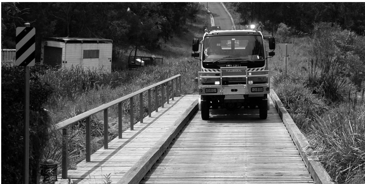
Property access should not restrict firefighting access. Bridge loadings should be clearly marked.
