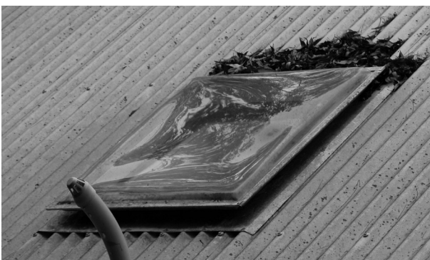
Poor design does not aid flushing of debris
