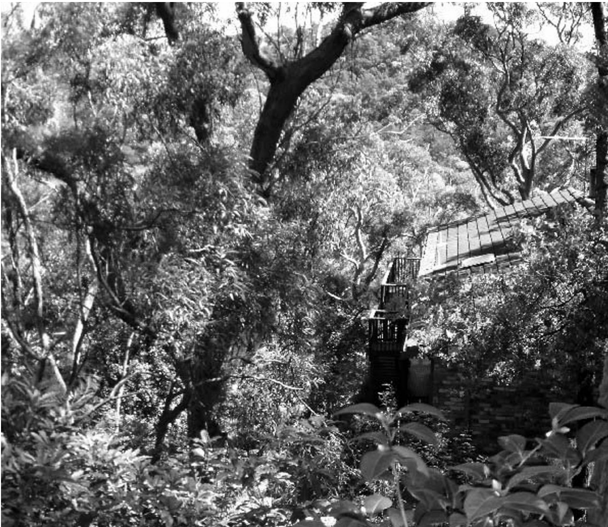
Some past planning practices have provided no effective protection to life and property in the event of a severe bush fire.
