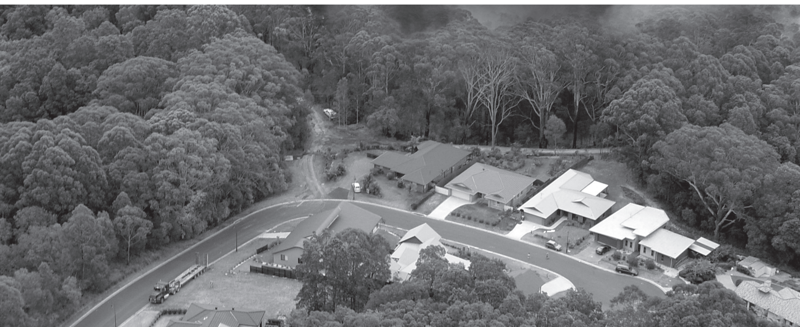
Perimeter roads should be the normal arrangement for urban areas and not perimeter fire trails.
