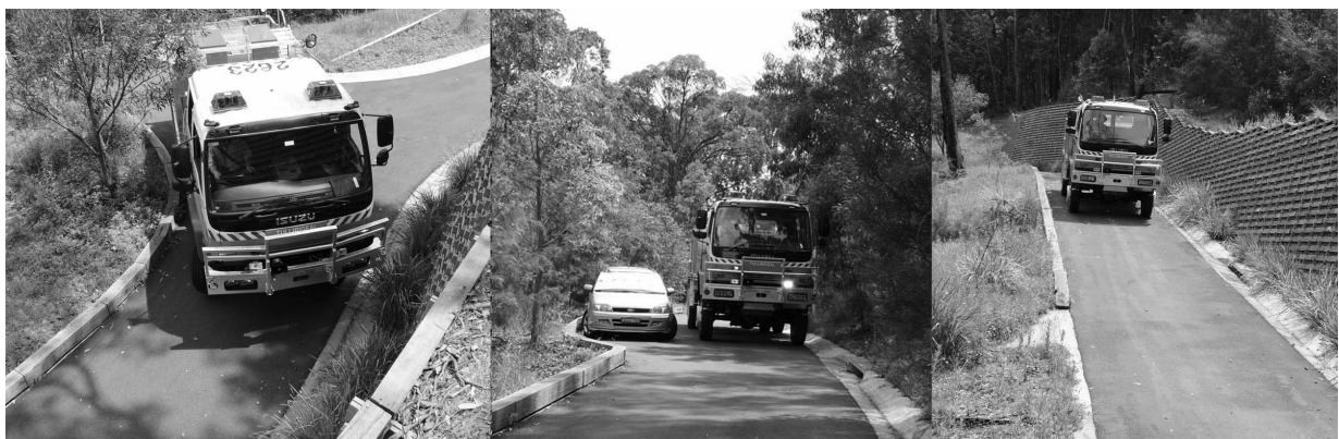
Examples of public road access arrangements that do not facilitate bush fire fighting.
