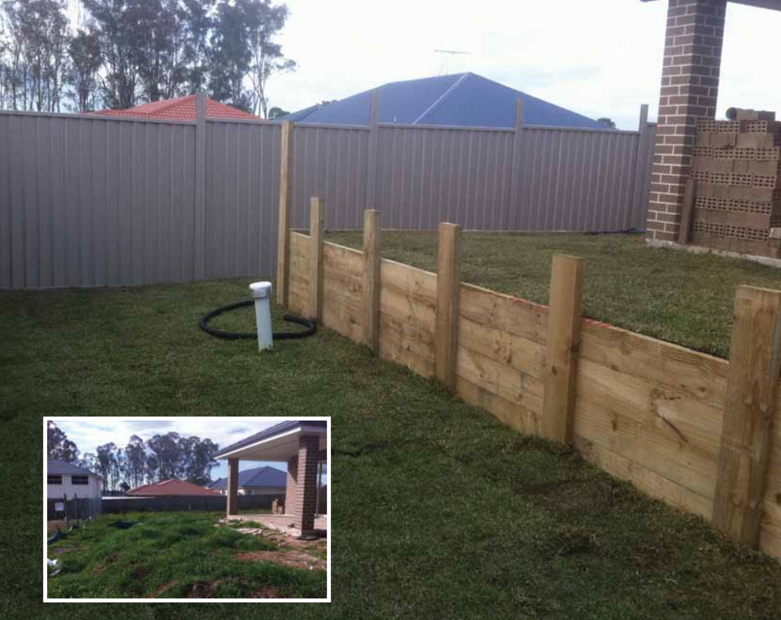
INSET (BEFORE): With the house finished and Katherine still in hospital, Troy had very little opportunity to consider the landscaping. AFTER: Long days and an enormous effort by everyone transformed the backyard for Troy and Katherine. Photos by Justin Back
